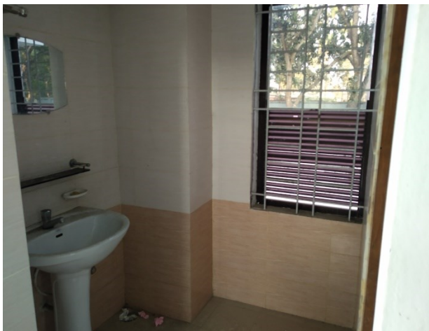
Pic 24: Wash Room Facilities
