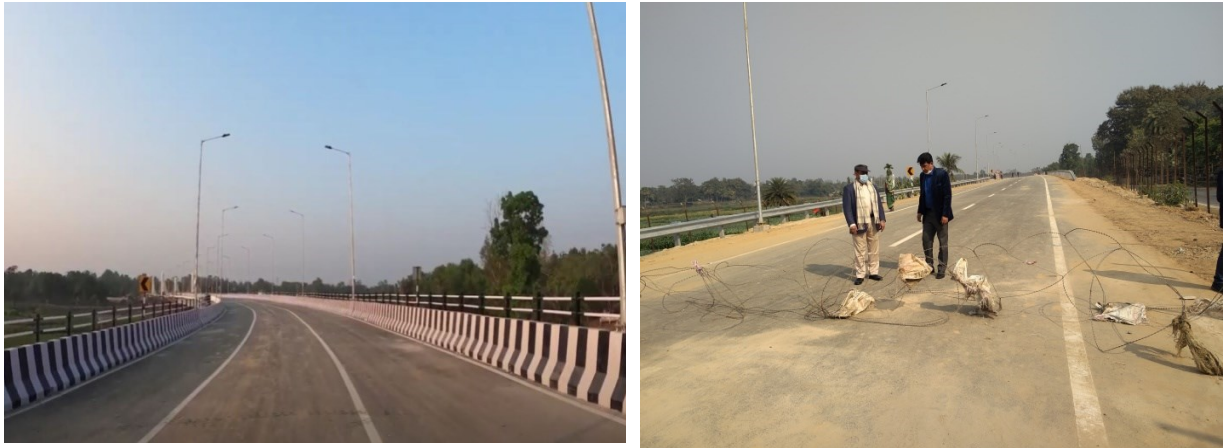
Pic 43: The Indo-Bangla Maître Bridge 1 over the River Feni
