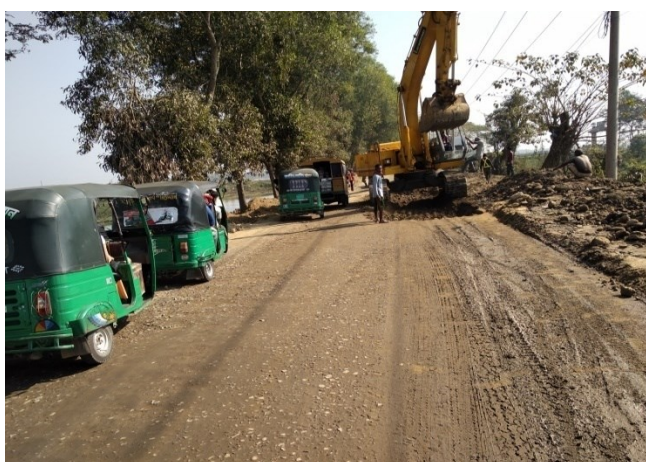
Pic 41: Road Improvement Activities
