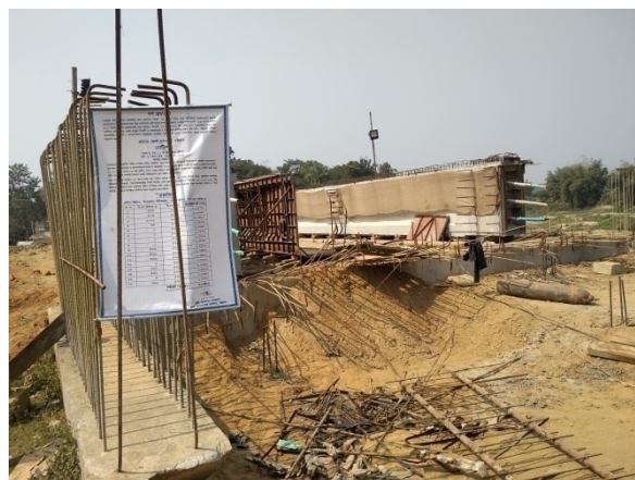
Pic 44: Road Improvement Activities
