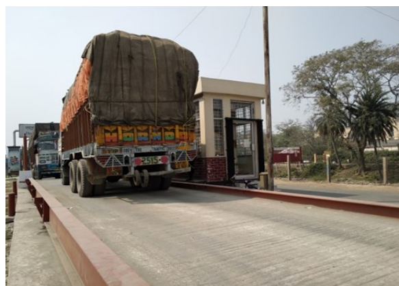
Pic 6: Weighbridge Scale Facilities
